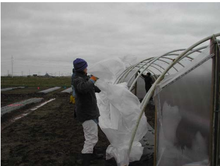
Figure 7. The Plastic As It Is Thrown Over the House.
